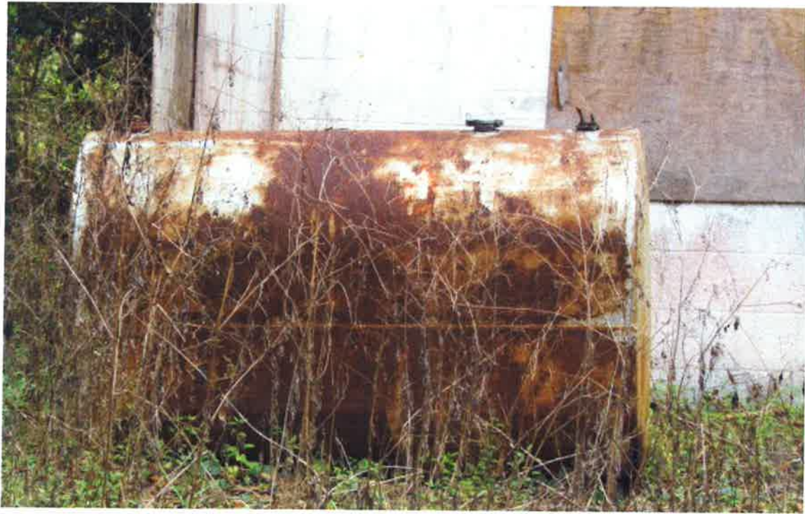
Plate 24 A view of an aboveground storage tank (AST) within the subject property.
